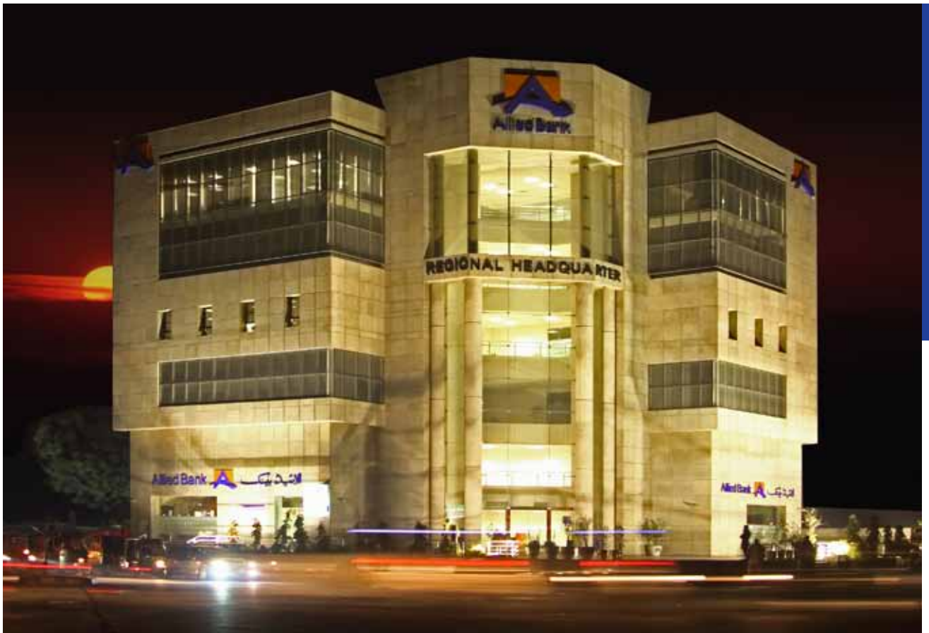
Regional Headquarter, Faisalabad
